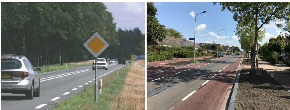
Fig. 5 On the left a distributor road with double-line center markings and on the right an access road with red asphalt marking the bike path
