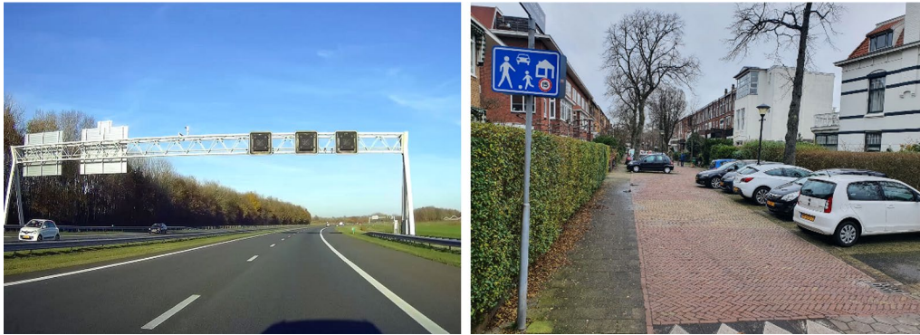
Fig. 4 Two types of roads which can be considered to be self-explaining. On the left a typical Dutch motorway with defining features for fast driving such as wide lanes, smooth asphalt, an emergency lane, guard rails, overhead lane control signs, no sharp curves and a lot of preview. On the right, a typical Dutch woonerf (also known as “shared space”) designed for slow driving (maximum speed 15 km/h) with defining features such as physical barriers, shared and paced space and landscaping and street furniture
